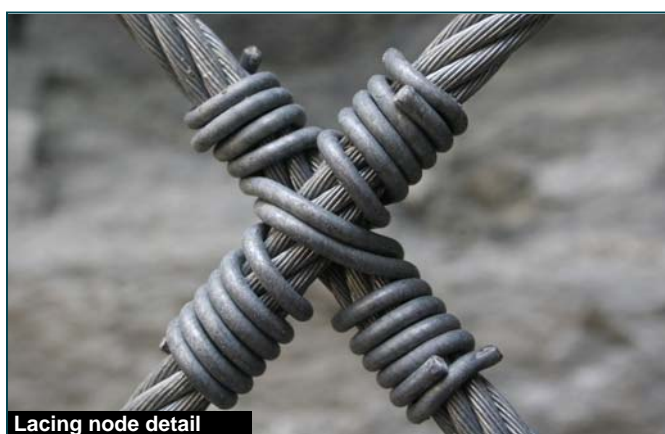
Lacing node detail
