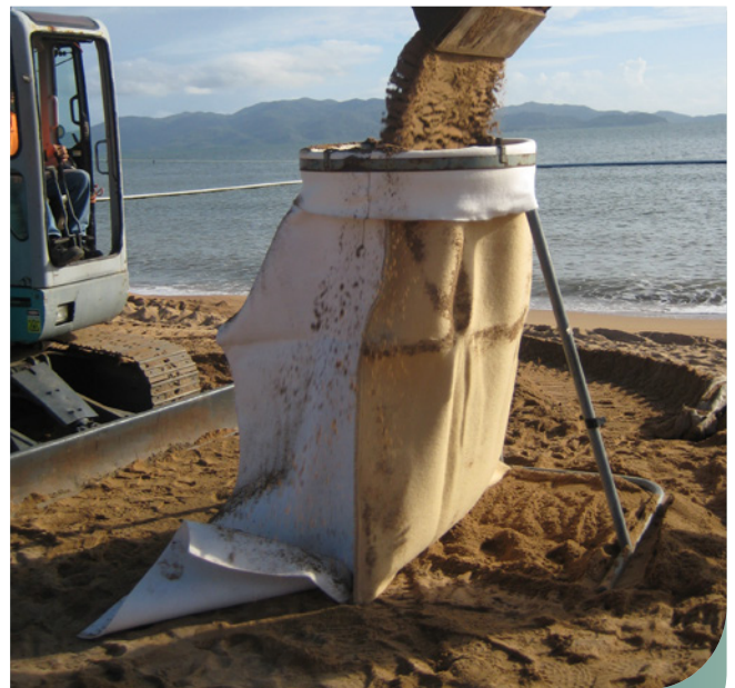
Figure 3. Filling sand container
