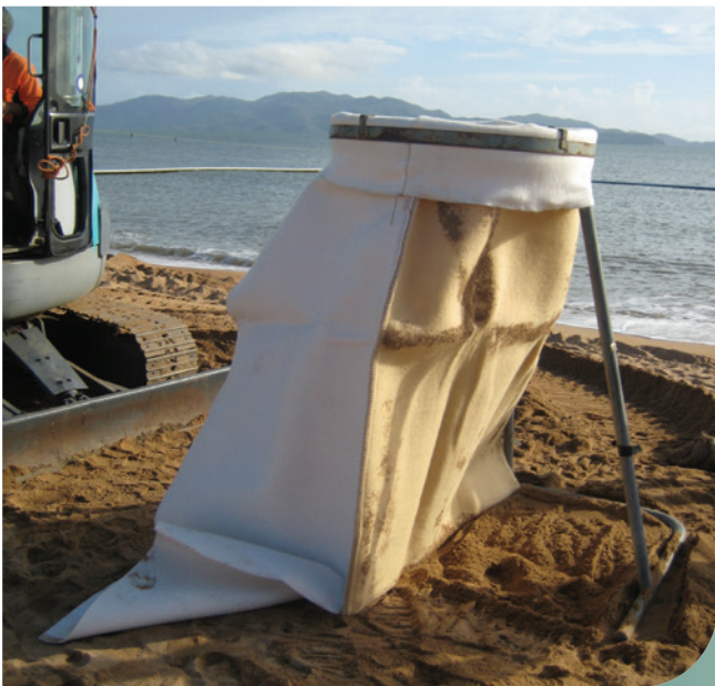
Figure 2. Securing sand container
