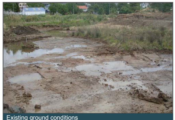
Existing ground conditions
