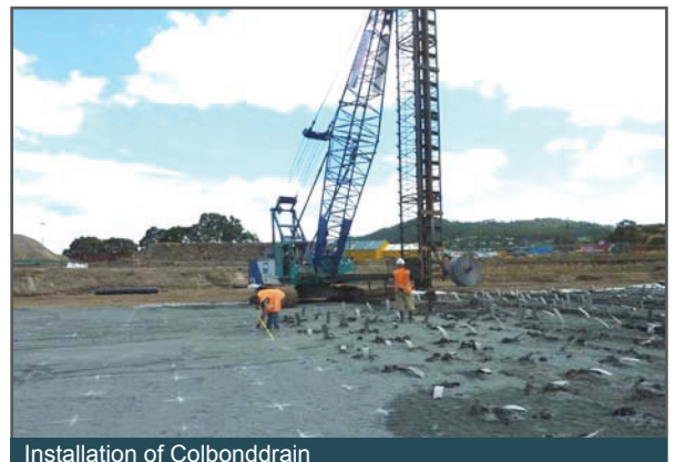
Installation of Colbondrain
