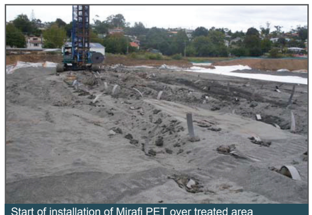
Start of installation of Mirafi PET over treated area
