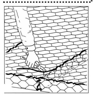
Place the fill material, by hand or mechanically, in the compartments, starting at the bottom if on a slope. The fill should be a hard, durable stone, in size between 80mm and two-thirds the thickness of the mattress, but generally no greater than 200mm.
