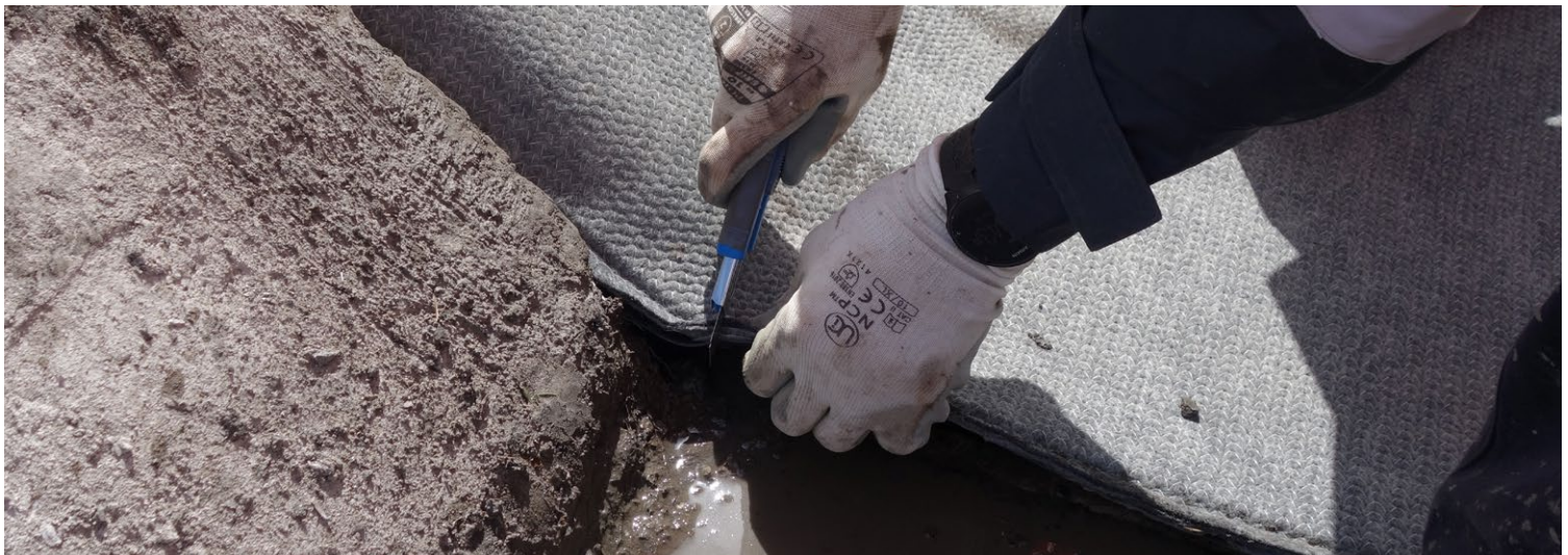
Figure 3. Cutting CCX™ using a 'snap-off blade' utility knife
