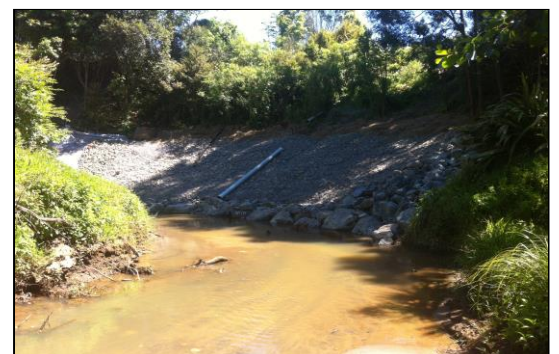
End of 130m of Reno Mattress protection
