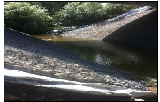
Below River Road Bridge
