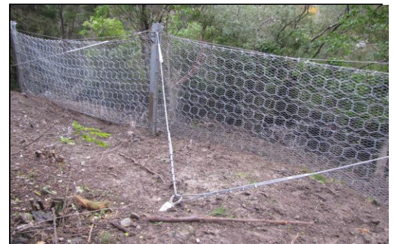
2000kJ Energy Rating Barrier Fence
