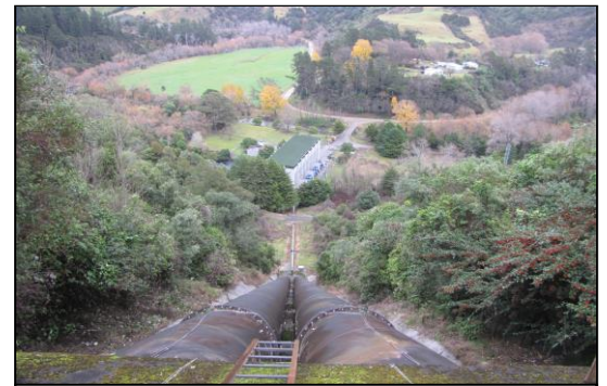
Existing Penstock line needing protection
