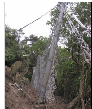
2000kJ Energy Rating Barrier Fence
