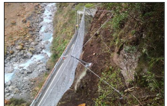
Rockfall hybrid fence (Photo courtesy of Abseil Access Ltd)
