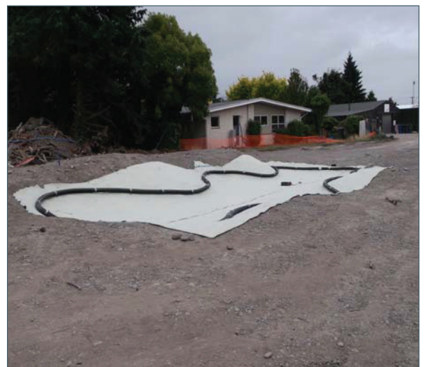
During construction, Jan 2013
