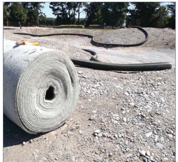
Preparing site for BunkerMat installation, Jan 2013
