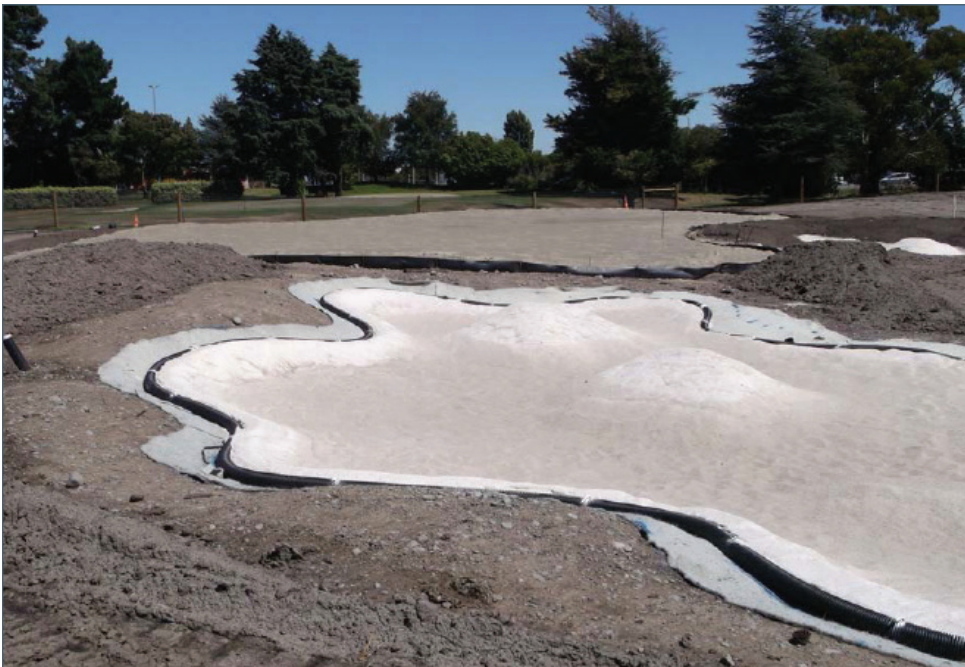
Preparing site for BunkerMat installation, Jan 2013
