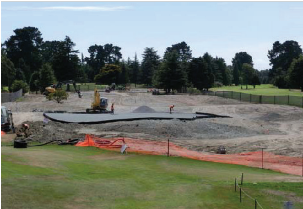
Preparing site for BunkerMat installation, Jan 2013
