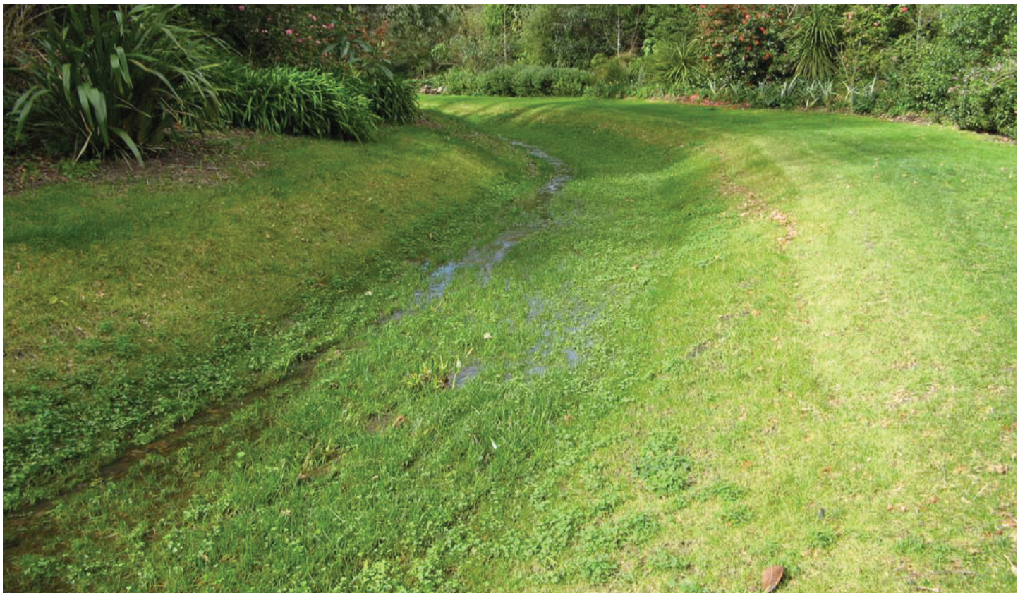
Completed vegetated stream
