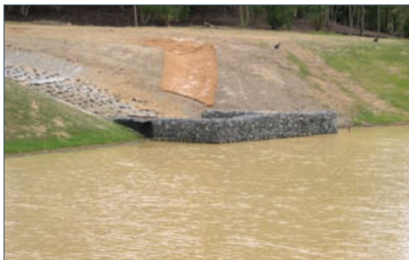
Gabion outlet structure at sediment pond
