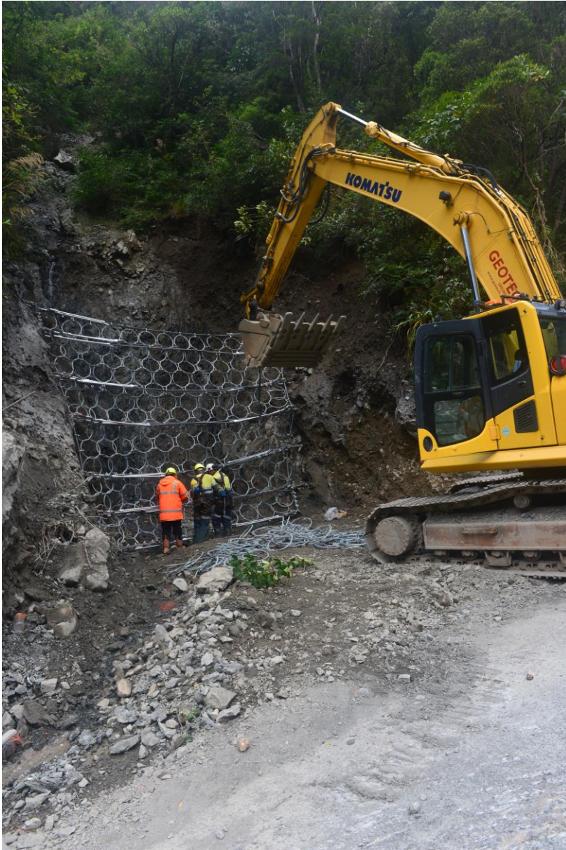
Debris Flow Fence near completion (Photo courtesy of Geotech Ltd)
