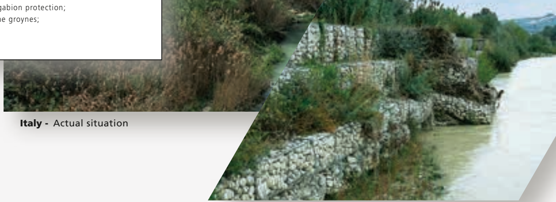
Microhabitat check schematisation (Research on the environmental effects by rivers sides with Gabion and Reno® mattresses)-Italy 1993-1994.
