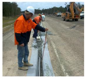
Because non-woven geotextiles such as Filterwrap are highly porous, water can pass freely while fine particles are prevented from moving through. This allows Filterwrap to be used where drainage or control of groundwater is an issue.
