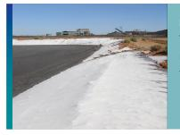
Texcel restricts the migration of fine soil particles from a soil mass while remaining permeable to water movement at a rate at least equivalent to the permeability of the retained soil.
