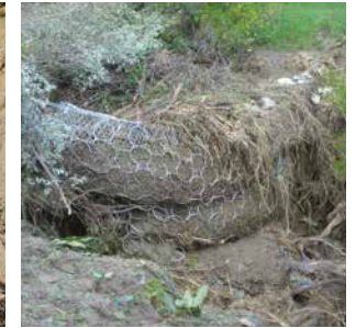
4 Debris Flow & Shallow Landslides
