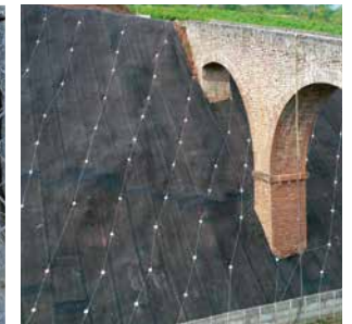
6 Soil Nailing and Surface Protection
