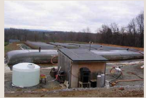
Geotube® dewatering cell
