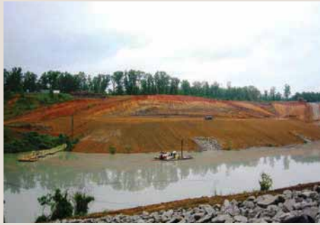
Reclaimed site after dewatering
