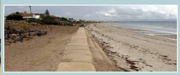
These medium sized sand containers are used typically in sea walls and groyne structures where sites experience mild conditions. Also often used in emergency works and temporary structures. Although the product is available in both standard and vandal deterrent materials, it is highly recommended where there is public interaction or chance of impacting debris that the vandal deterrent material is selected. Scour flap containers are also available in this size.
