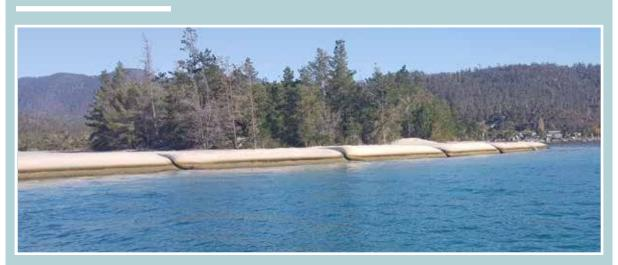
Elcorock Mega containers are engineered sand filled tubes that offer excellent performance in durability, robustness and usability providing the designer, contractor and end user a product that is capable of withstanding some of the harshest conditions.
