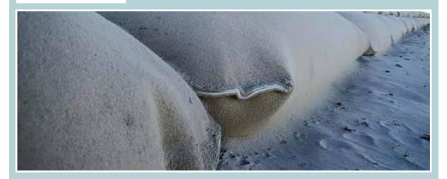
Due to the increased fill port on these 1.2m<sup>3</sup> containers, they tend to be quicker to fill which makes them ideal in emergency or temporary type structures.
