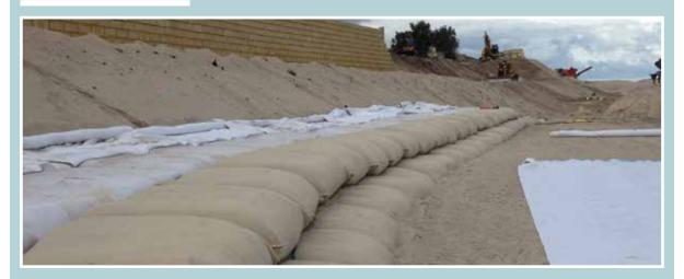
These large hopper filled sand containers are used in revetments and groynes, due to their large size and high stability, even under the harshest of conditions.
