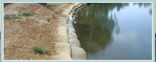
These containers are the smallest of the Elcorock sand containers. Generally used on inland protection works, stream protection and small on shore structures in very mild conditions. Easily filled with little mechanical equipment required for installation and filling makes the containers suitable for community groups or land owners.
