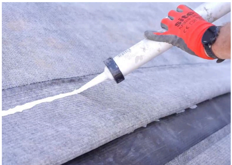
Overlapping layer of CCX-B™ sealed with adhesive
