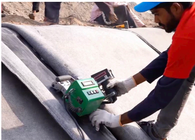
Overlapped layers of CCX-B™ thermally welded
