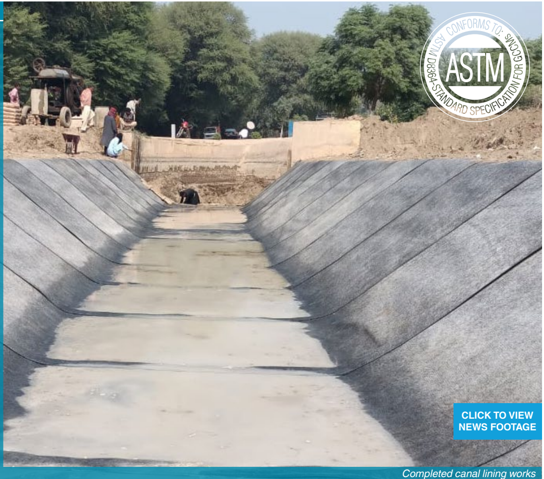
Completed canal lining works
