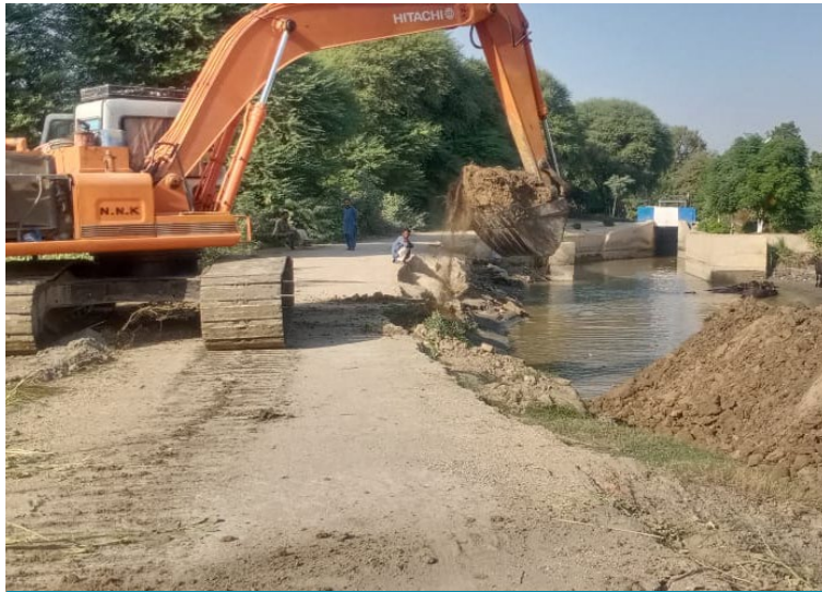
Existing canal backfilled in preparation for profiling
