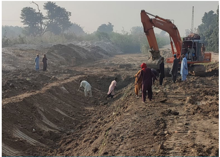
New profile excavated for CCX-B™ install
