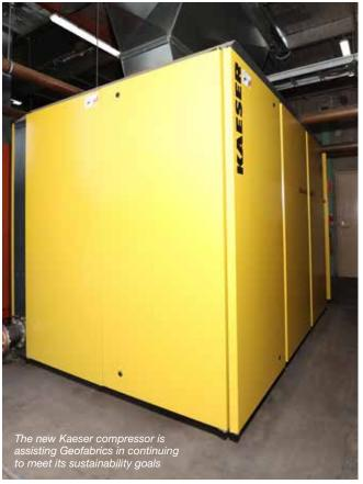
Finally, an intelligent component layout ensures even greater energy efficiency: for example, all service and maintenance points are within easy reach and are directly accessible from the front of the unit. This not only saves time and money when performing service work, but also maximises compressed air system availability.
