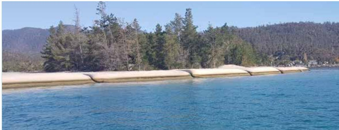
Elcorock Mega containers are engineered sand filled tubes that offer excellent performance in durability, robustness and usability providing the designer, contractor and end user a product that is capable of withstanding some of the harshest conditions.
