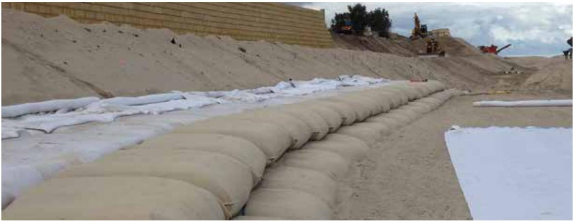
These large hopper filled sand containers are used in revetments and groynes, due to their large size and high stability, even under the harshest of conditions.
