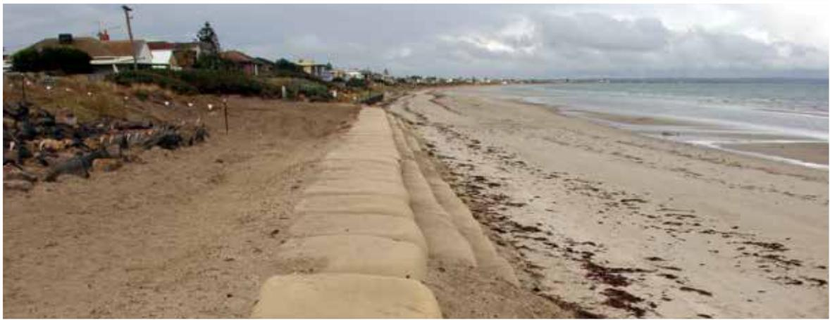
These medium sized sand containers are used typically in sea walls and groyne structures where sites experience mild conditions. Also often used in emergency works and temporary structures. Although the product is available in both standard and vandal deterrent materials, it is highly recommended where there is public interaction or chance of impacting debris that the vandal deterrent material is selected. Scour flap containers are also available in this size.
