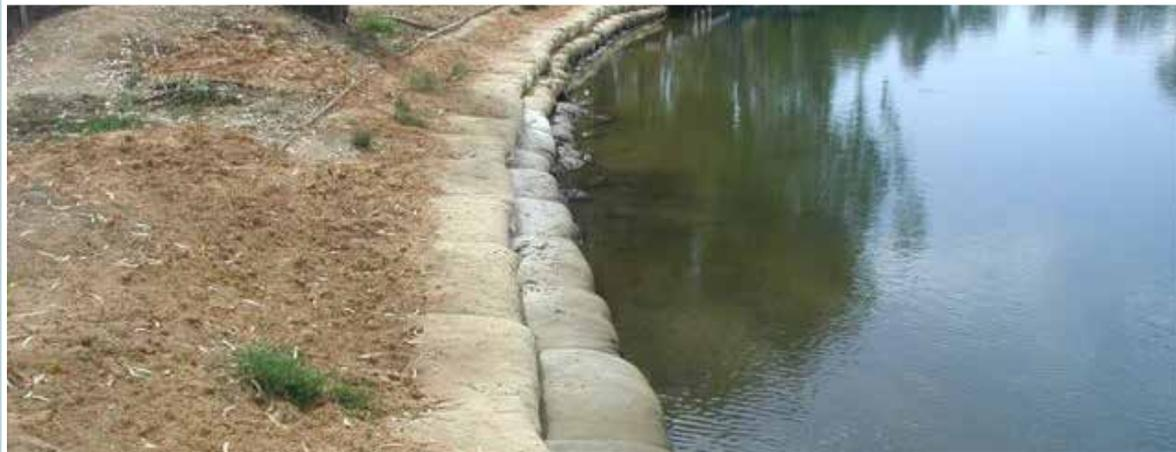
These containers are the smallest of the Elcorock sand containers. Generally used on inland protection works, stream protection and small on shore structures in very mild conditions. Easily filled with little mechanical equipment required for installation and filling makes the containers suitable for community groups or land owners.
