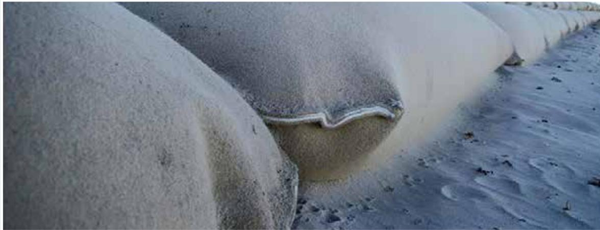
Due to the increased fill port on these 1.2m<sup>3</sup> containers, they tend to be quicker to fill which makes them ideal in emergency or temporary type structures.
