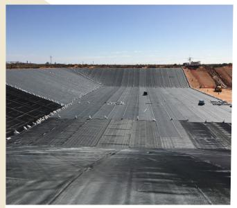
Geocomposite drain and conductive geotextile being installed
