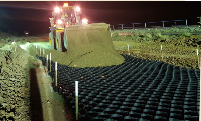
The Geoweb was then infilled with a capping layer material
