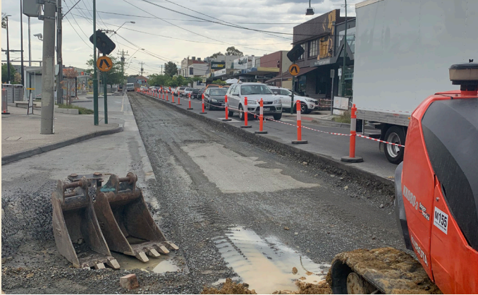
Soft subgrade after first attempt of compaction prior to the bidim and Tensor TriAx Tx160.
