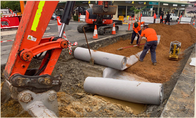
Additional excavation and install of bidim separation.
