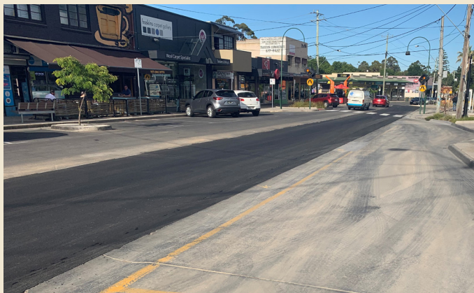
Completed road and bus turn-outs.
