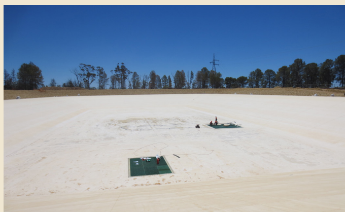
Pictured is the 30 year Liner: Ethylene Interpolymer Alloy (EIA) Oasis 1.14 mm.
