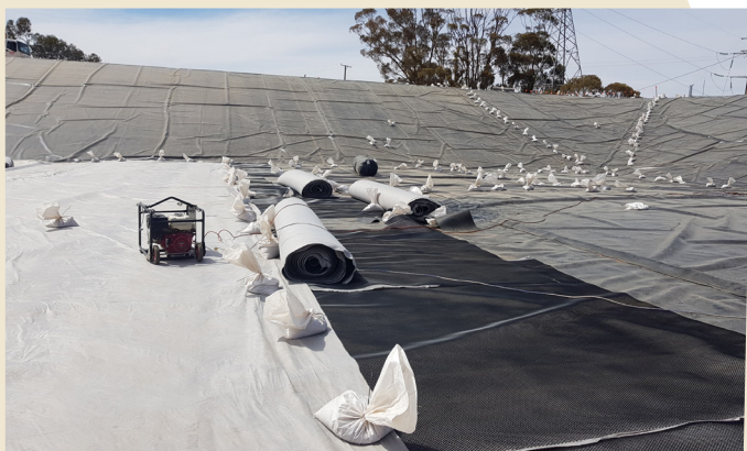
A64 Geotextile cushion layer over the drainage layer.
