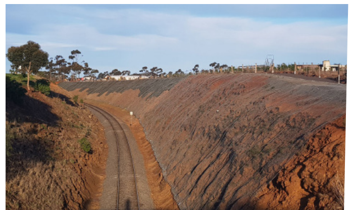
Completed Steelgrid rockfall mesh system.
