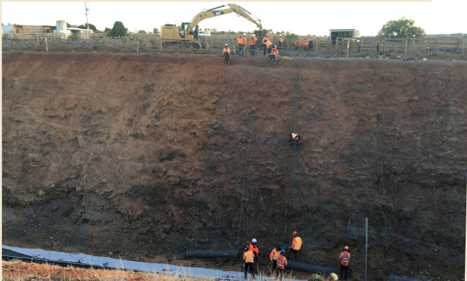
Coleman Rail installed the Steelgrid with rope access techniques.
