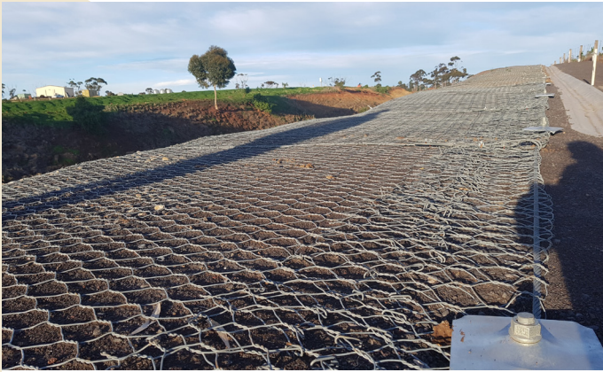
Top anchoring detail using Galvan coated steel wire rope and the Steelgrid system anchor plate.
