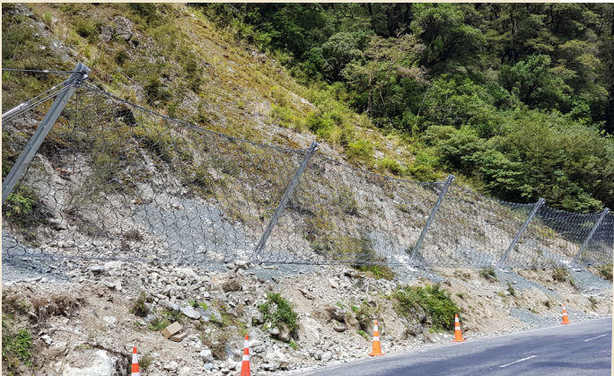
Completed 2000 kJ Maccaferri RMC200A certified fence.
