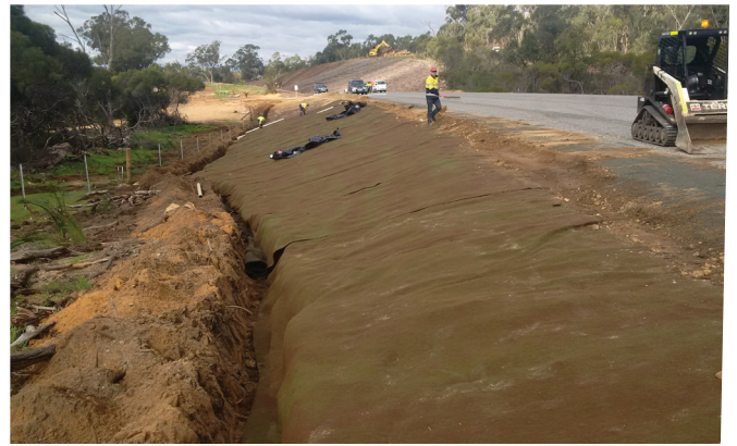
During installation in 2014
