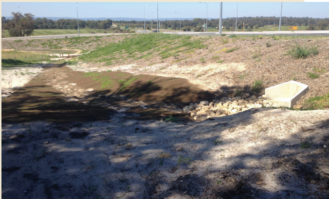
Completed install at drain outlet and 80 m slope
