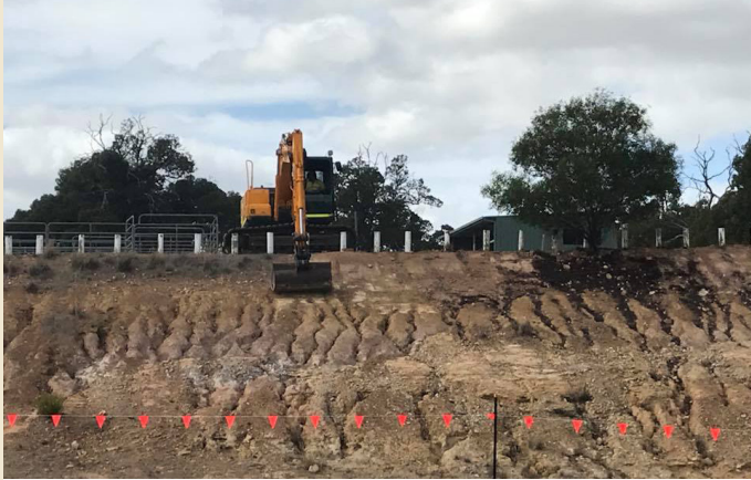
Severe rill erosion from surface run off on the slopes around the hockey field.
