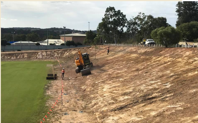
During slope re-profiling in preparation for the Grassroots.
