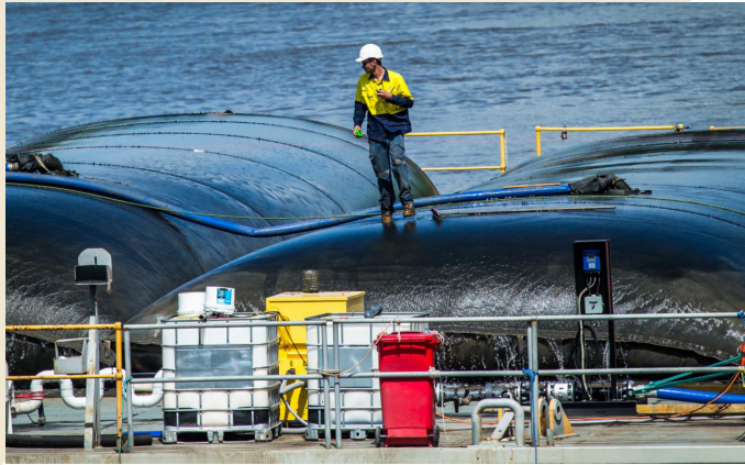
Geotube® units while dewatering.
