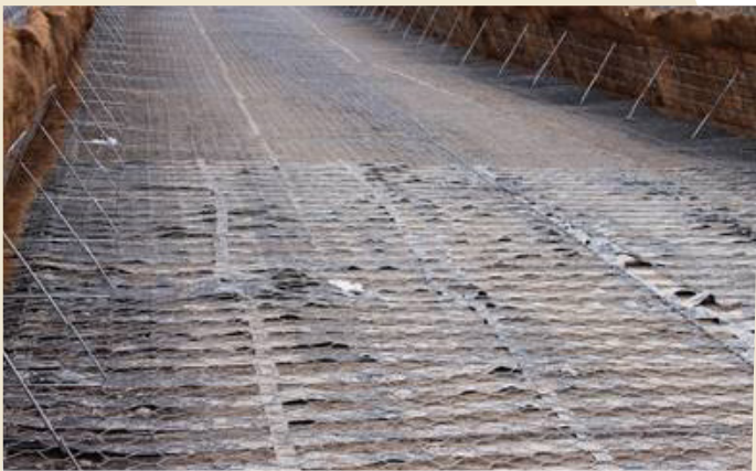
Paralink 200 geogrid as primary reinforcement.
