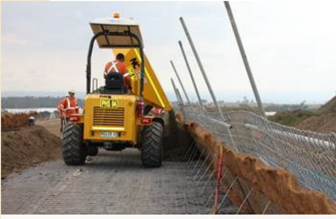
Placing vegetative soil behind the face of the wall.
