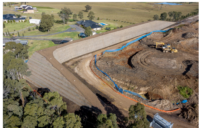
Aerial photo of completed bund.
