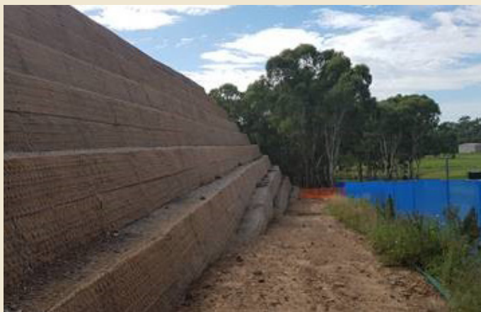
45 degree face achieved by stepping back every second layer.
