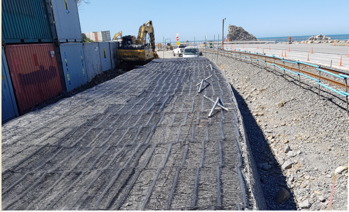
Tensar RE560 uniaxial geogrid in lower part of bund.
