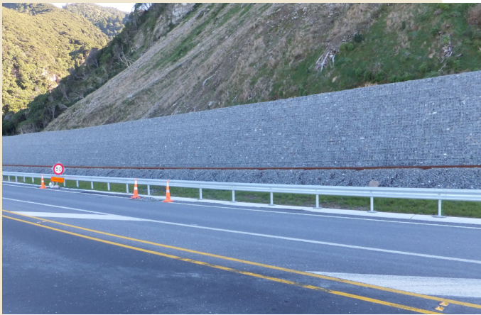
Hand placed rock in front face.
