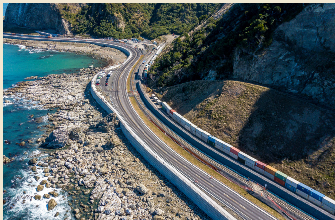
The longest Maccaferri Green Terramesh rockfall bund in the world.
