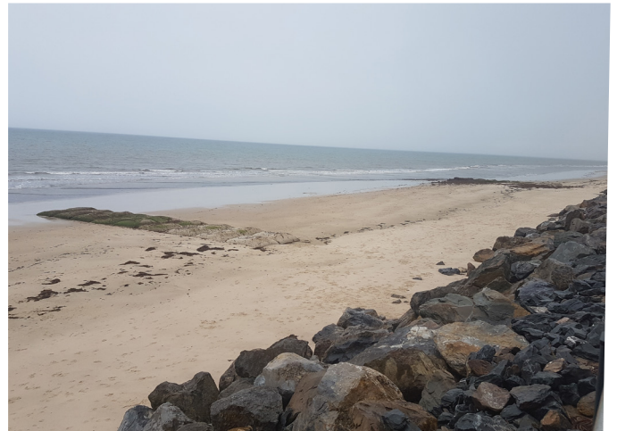
Elcorock Groynes at the end of 2018 after Winter. Historically, the beach at this time of the year was near non-existent, however the bags are working extremely well, capturing sand and thus building up the beach.
