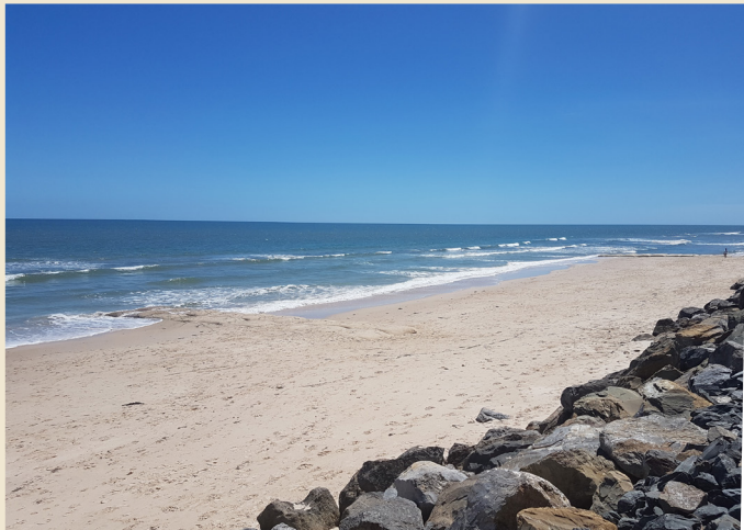
Completed Elcorock groynes blending to the beach in 2017
