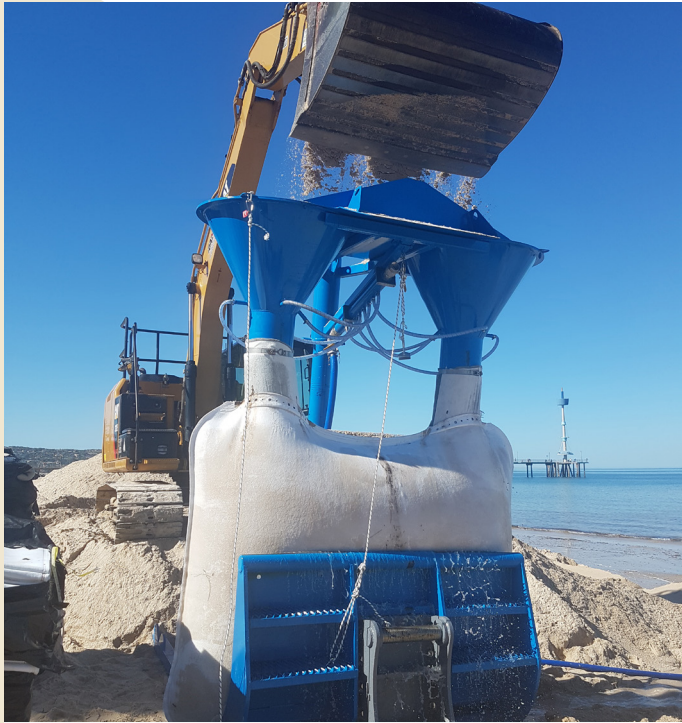
Filling the Elcorock sand containers
