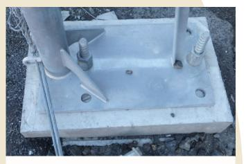
Up slope anchors not required
