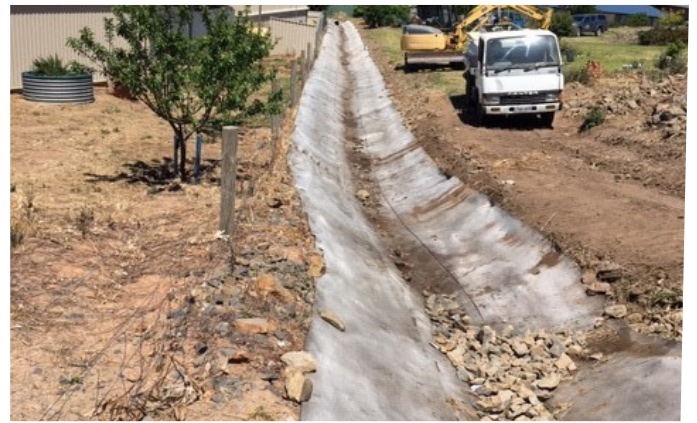
Hydrated and finished Concrete Canvas swale lining.
