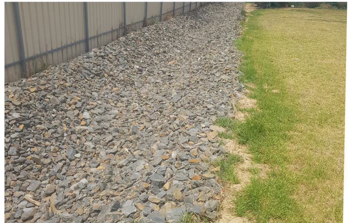
Completed project covered in rock to slow water flow.
