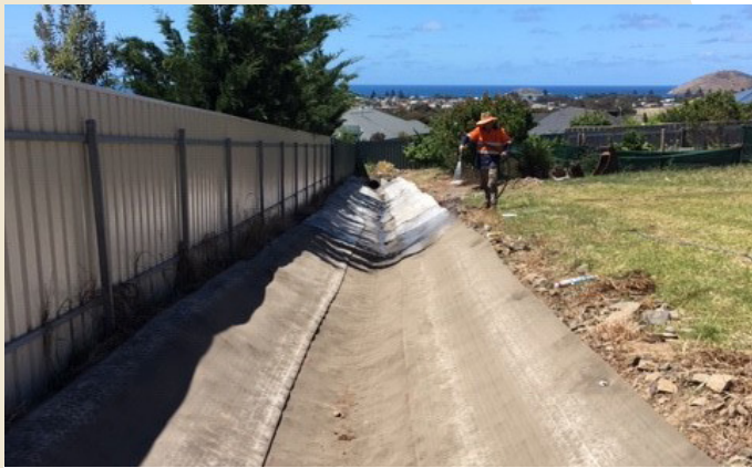
Laid Concrete Canvas prior to hydration.
