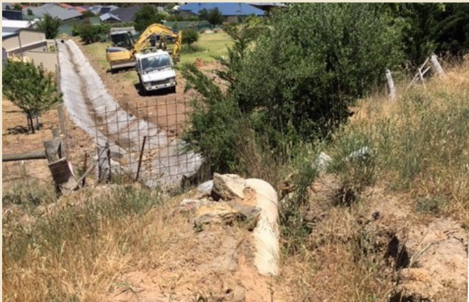
During laying of Concrete Canvas viewed from the top of the swale.
