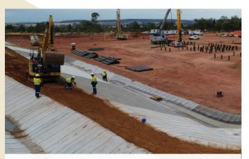
Concrete Canvas was the best option to fill the brief of both channel lining and erosion control.
