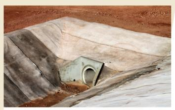
Concrete Canvas was laid transversely after the removal of vegetation on cut batters in drains.
