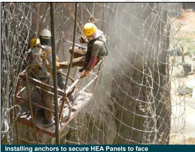
Installing anchors to secure HEA Panels to face
