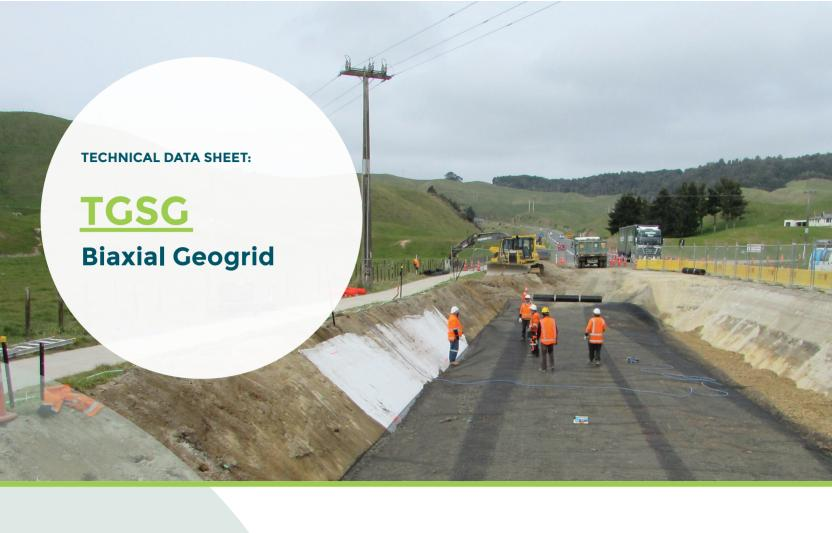
TGSG biaxial geogrids are used for the reinforcement of soils and aggregates in construction of road pavements, hardstands, working platforms and reinforced foundations.
