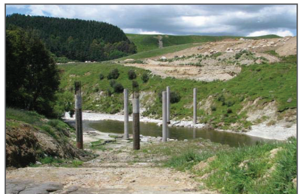
Bridge prior to construction with piers installed, Feb 2009
