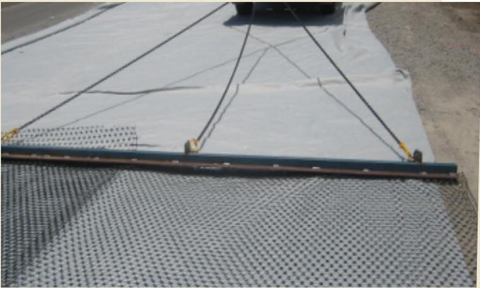
Tensioning the bar to control the movement and stiffness of the grid.
