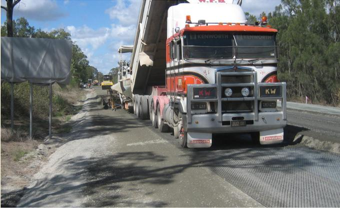
Laying granular fill over the TX geogrid.
