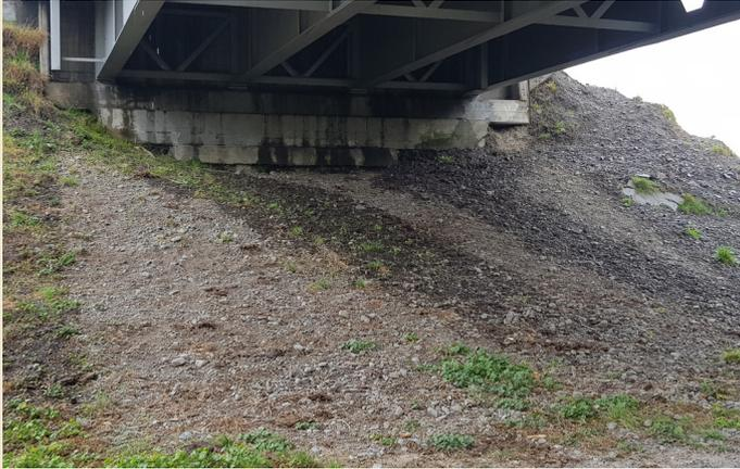
Eroding Bridge Abutment before the Green Terramesh installation.
