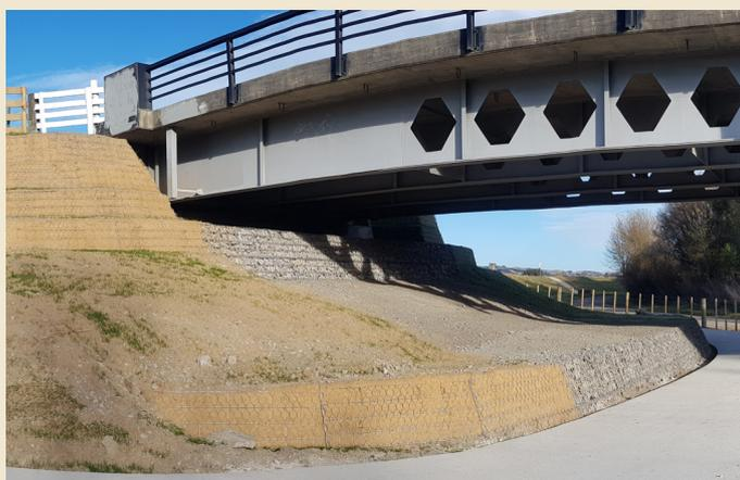
Completed Green Terramesh structure with both vegetation and rock face.
