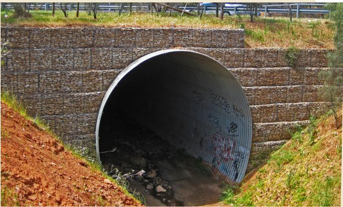
The Terramesh structure upon inspection in 2008, nearly 20 years after installation.
