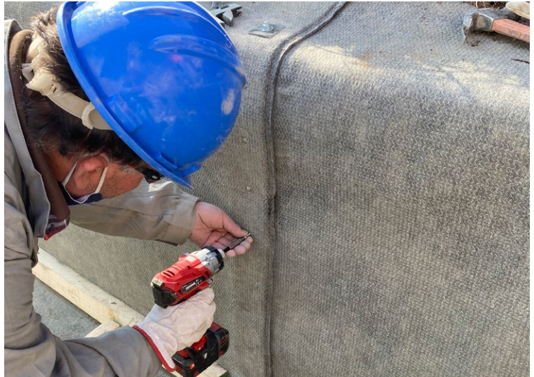
Screws are being fixed every 100mm
