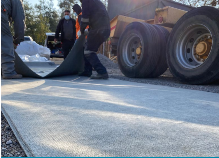
CCX-M™ being rolled out on site
