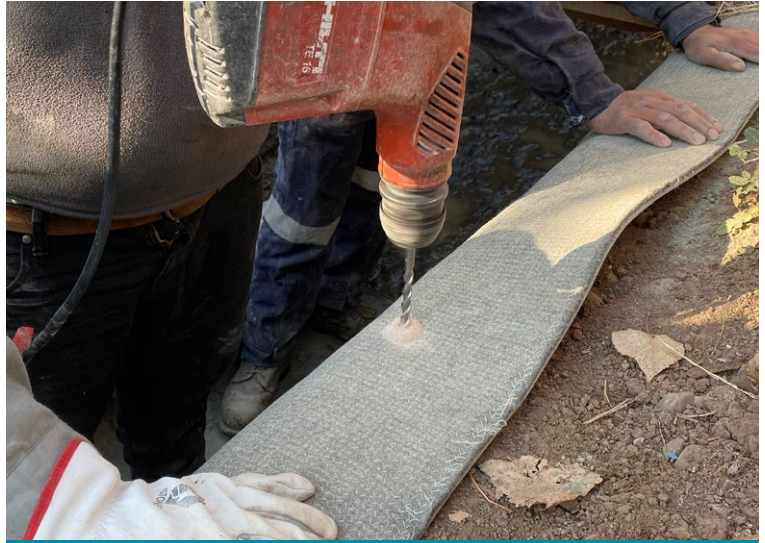
Holes being drilled for anchor bolt fixing
