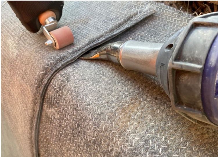
Thermal bonding overlap
