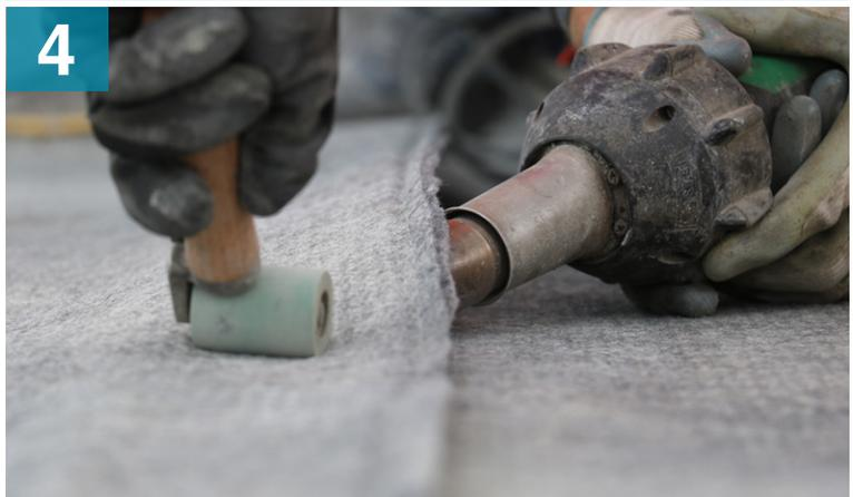
Thermally bonding overlapping layers of CCX™
