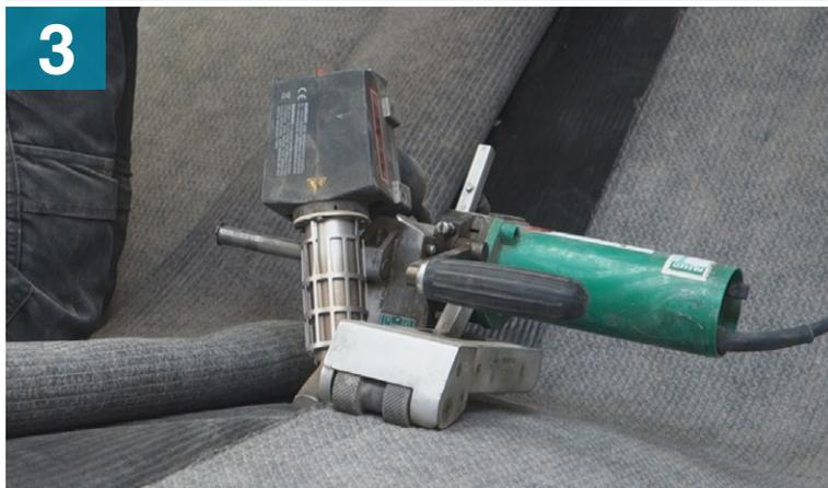
Thermal welding of CCX-B™ LLDPE backing
