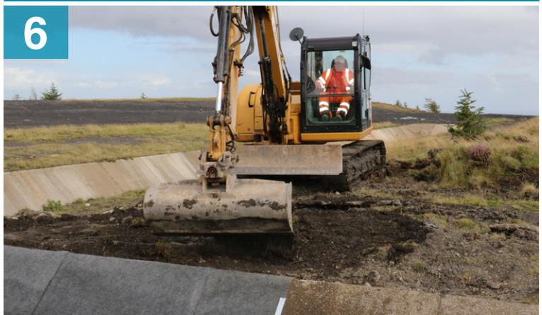
Backfilling anchor trenches to prevent ingress
